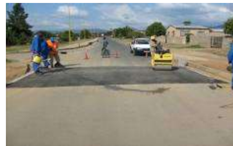
Construction of speed hump
