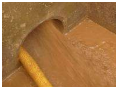
Cleaning of storm water pipe
