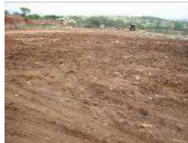
Umjindi Landfill Site with staff housing on the left hand side
