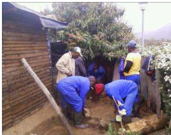
Repairing of midblock pipe
